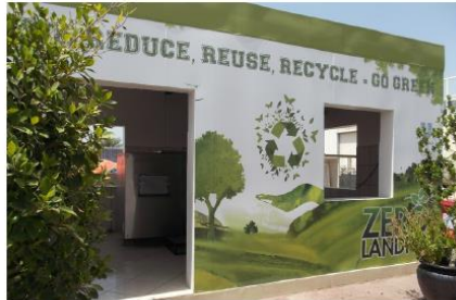
Site: Unilever Lipton Jebel Ali Factory Location: Dubai UAE Machine: GG100s Install Year: 2013 Publications: Unilever Press Release 2013
